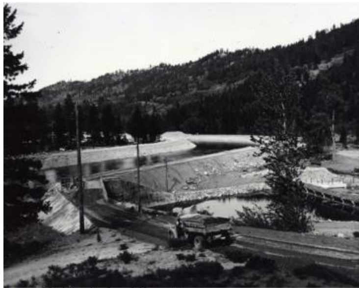
Leavenworth National Fish Hatchery construction in 1940. Photo courtesy of USFWS.
